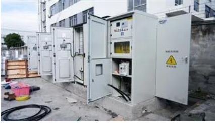
Flow batteries operating at remote sites in Latin America
