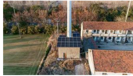
Environmental protection project uses 25kW outdoor photovoltaic
