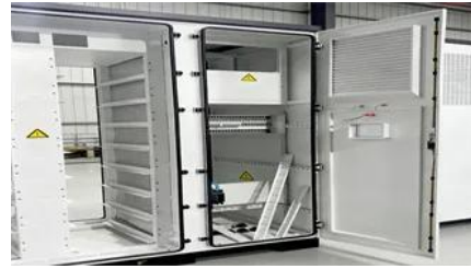
Solar container lithium battery for energy storage in Guinea-Bissau
