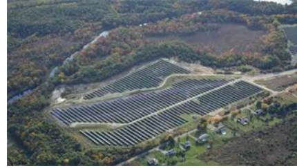
200KWH commercial energy storage system_Lithium Battery Storage
