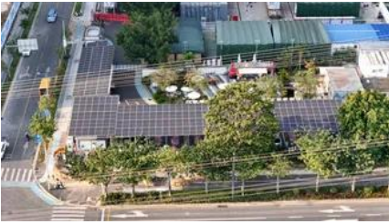
san marino outdoor telecom cabinet off-grid bulk procurement
