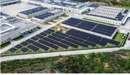
Swiss Zurich Power Plant Energy Storage Project Revolutionizing
