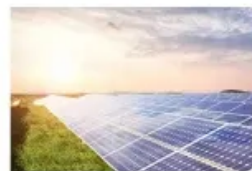
Energy Storage System
