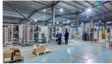
Niue EK solar container outdoor power 1 kWh , PABIANICE BESS
