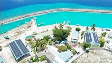
EBRD co-finances major renewable energy and battery
