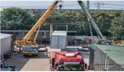
Weatherproof Outdoor Cabinets , Solar Battery Box Enclosures , Solar
