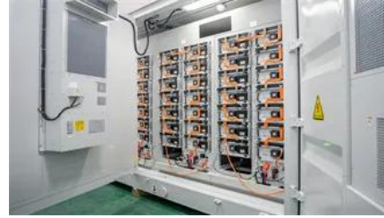
Somaliland solar container communication station inverter grid
