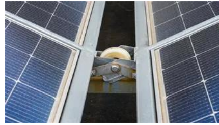
Common information of wind power in solar container.
